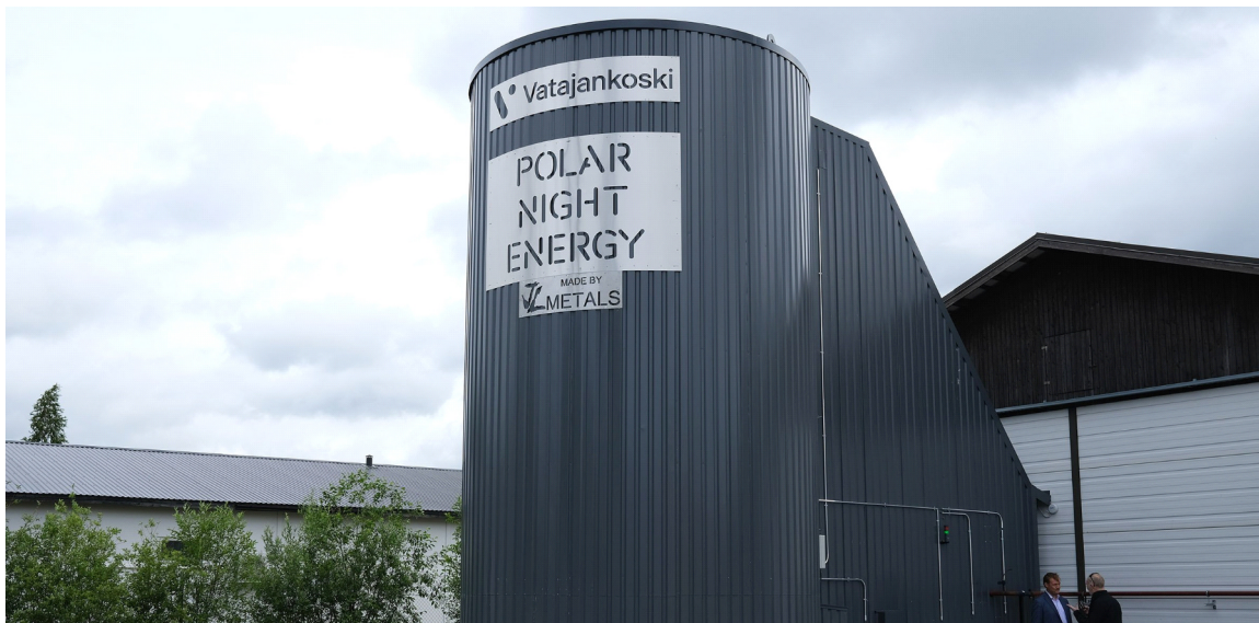
INNOVATIVE DESIGN/TECHNOLOGY EXAMPLES Right: Bambados Pool in Bramberg, Germany and Lippe Bad Lunen Pool in Lunen, Germany - both built to Passivehaus standards; below: Polar Night Energy Sand Battery in KanKaapaa, Finland
